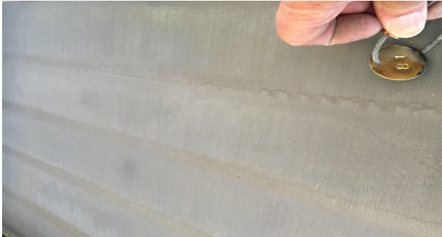
Figure 7 MDOT sample completely cleaned
